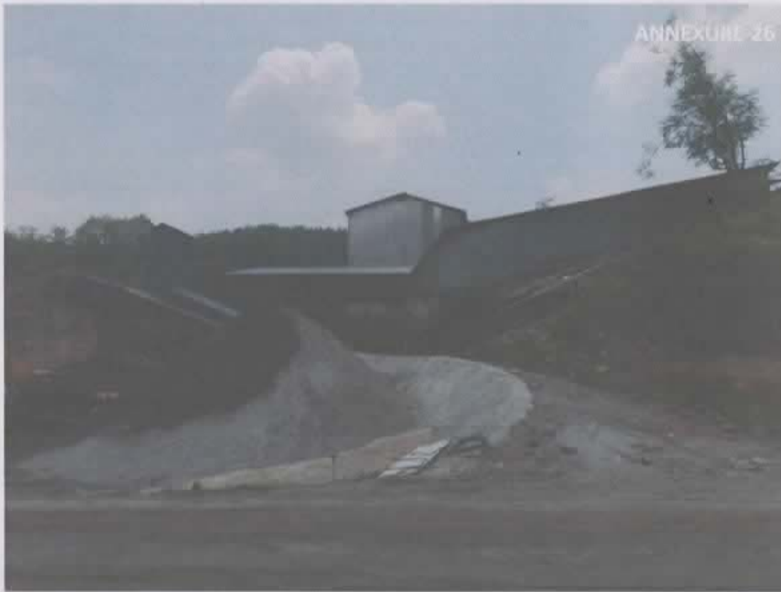
CRUSHER PLANT ACOUSTIC ENCLOSURES
