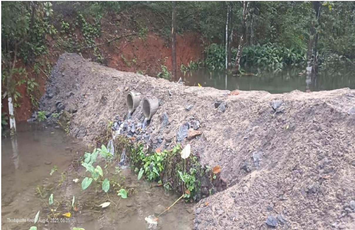
Drainage water sampling site
