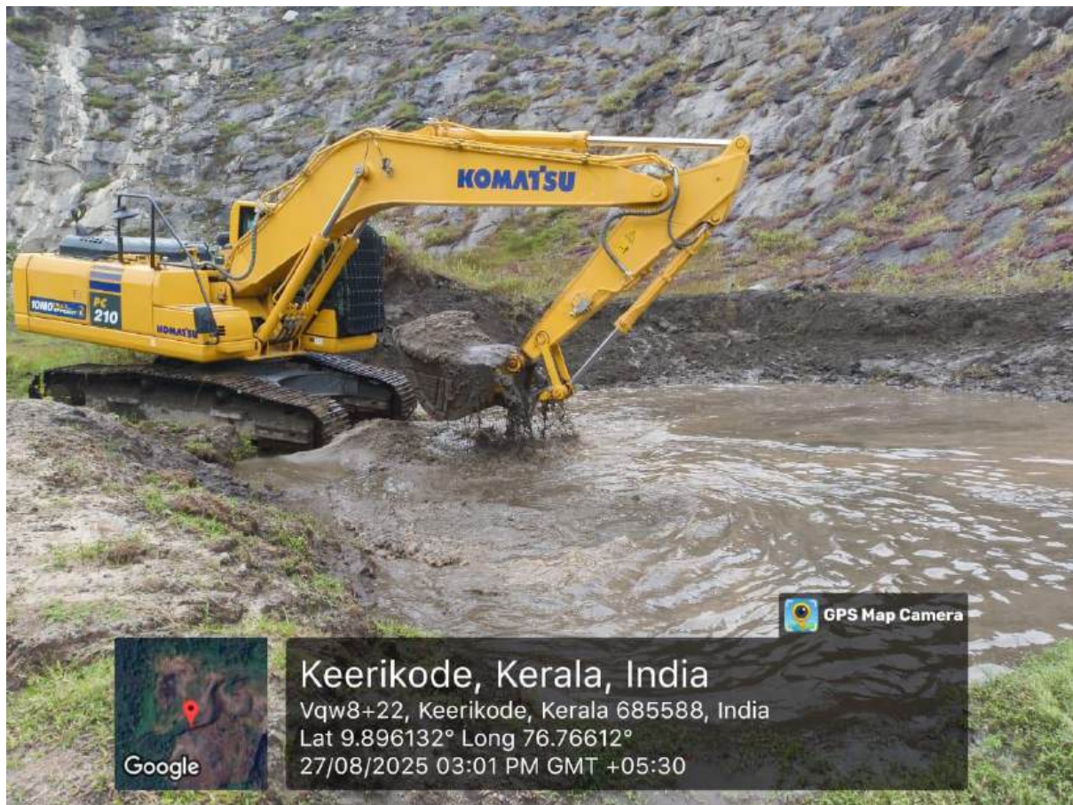
Settling Pond De-Silting
